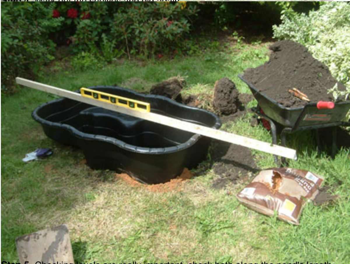
Step 5. Checking levels are really important, check both along the pond's length
