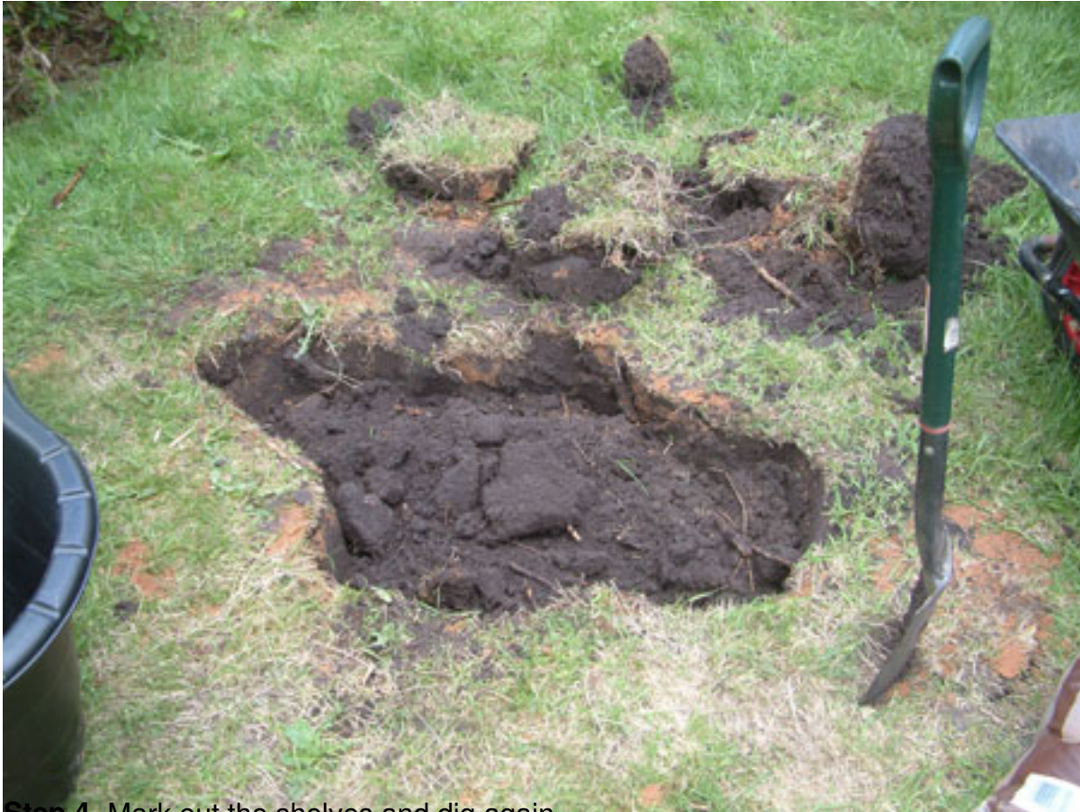
Step 4. Mark out the shelves and dig again
